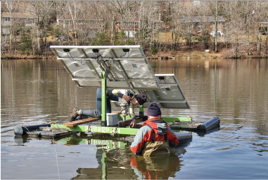
Fig. 7. Community volunteers set up Aquago for 2022 open water season on Oathill Lake in a densely settled neighbourhood of Dartmouth, N.S, Photo by Erle Hickey, with permission. More photos at https://www.flickr.com/photos/earle/51964726243/ The solar powered mixing device was installed in 2015. The deepest spot in Oathill Lake is 8.5 m, most of the lake is less than 5 m depth. Oxygen was depleted from 3 to 4 m depth to bottom over much of the summer season, now only in the deepest 1 to 1.5 m which occurs over a very limited area. Total P has declined significantly. The Aquago is one of a larger set of remedial measures introduced and maintained by the Oathill Lake Conservation Society. [46]
