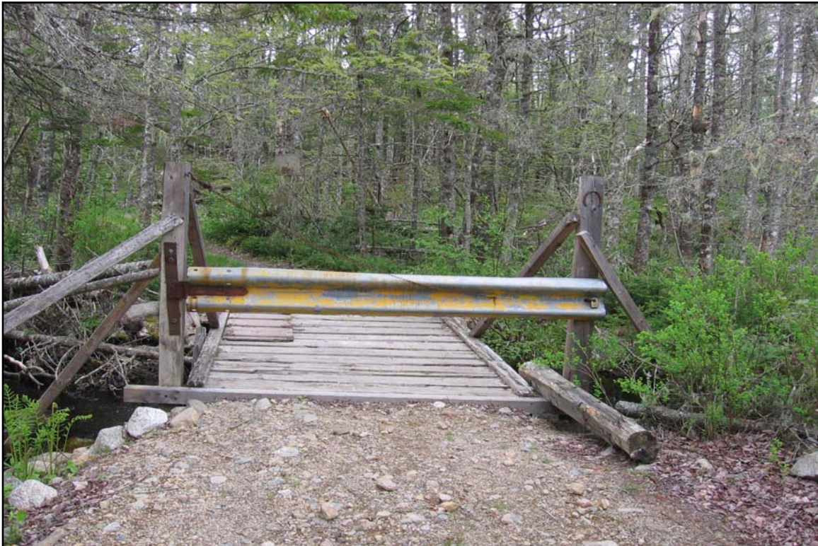
Photo 2: Road Access to Croucher Lake. Note Locked Gate (Private Property) and Unsafe, Narrow Bridge Preventing Vehicle Access
