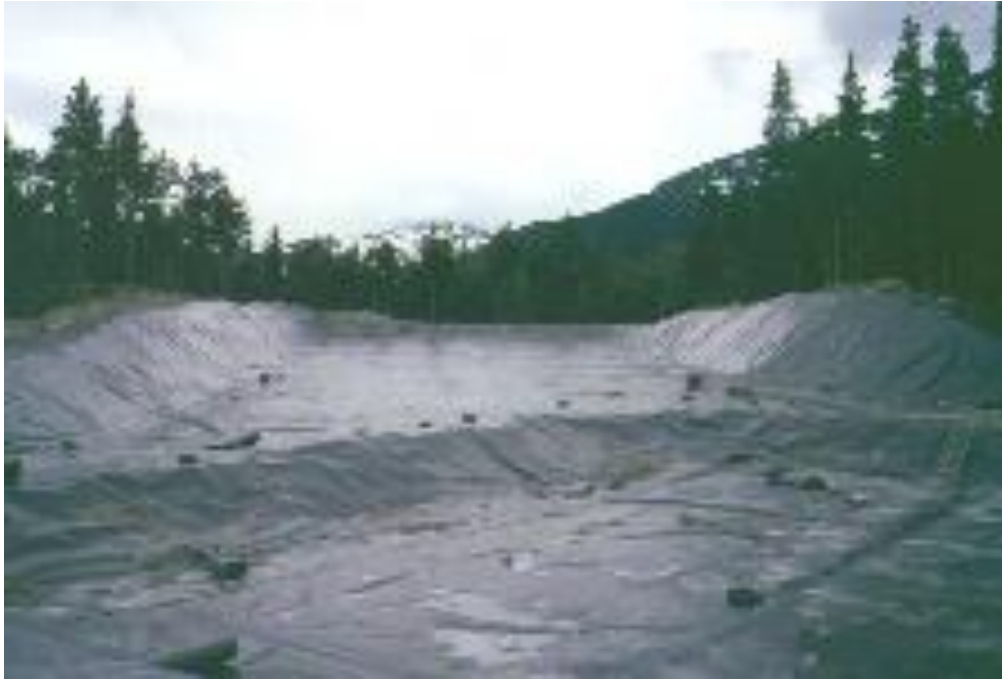
Figure 6.18 – A common geotextile fabric liner used in construction
