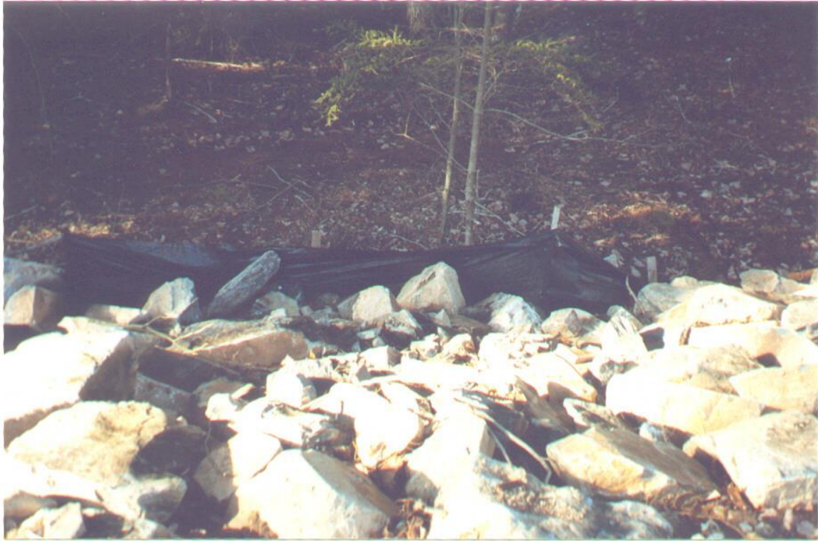
Figure 6.14 – A silt fence in use off the beach access road
