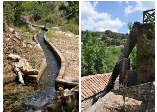
Figure 3: (a) the water channel and (b) the water charge reservoir
