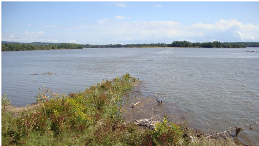
Photo 6: Crest of Great Dyke inundated at high tide
