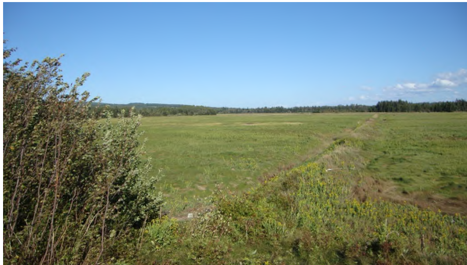
Photo 1: View of Great Dyke from west abutment, facing east
