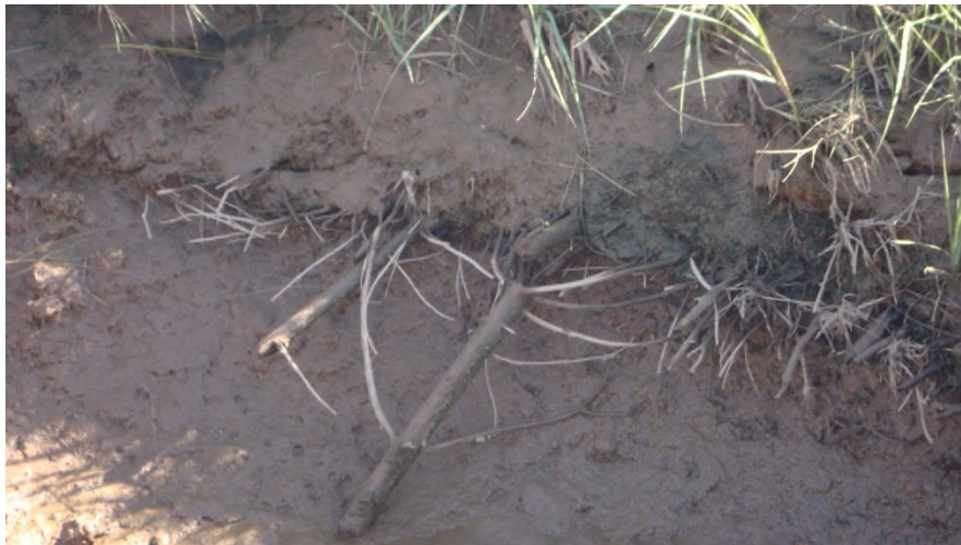
Photo 5: Use of brush layering beneath dyke fill near former location of aboiteau
